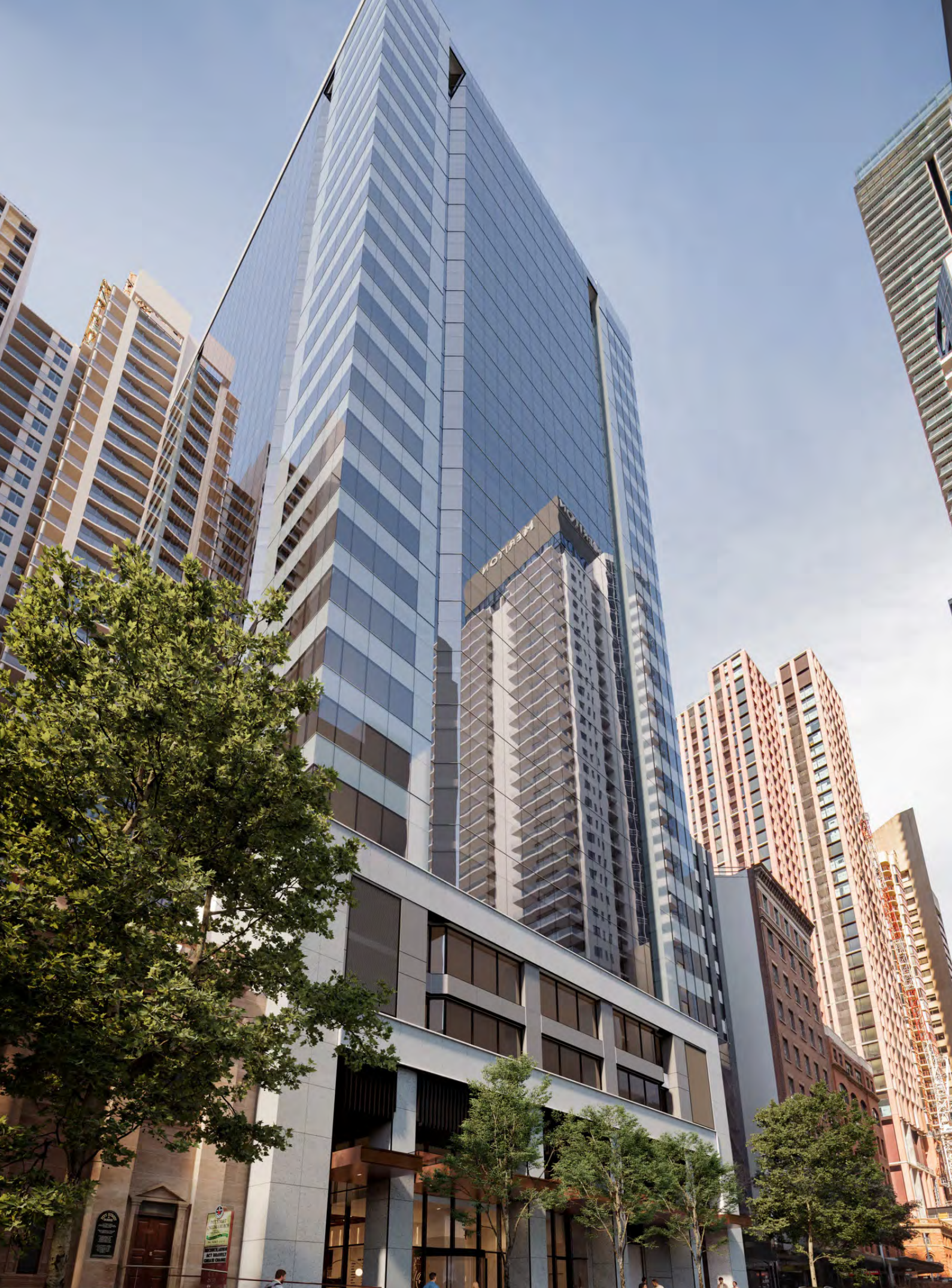
The full refurbishment of the former Defence Plaza at 270 Pitt Street (above) has just reached practical completion.
